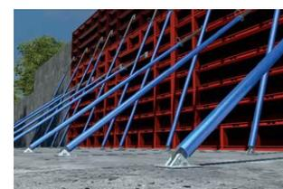
Formwork- and prop fixings
